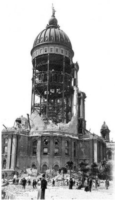
In 1908, San Francisco, California, experienced a very strong earthquake. The quake revealed that the buildings with internal steel structures held their shape and did not collapse. Brick buildings, on the other hand, were shaken apart.
